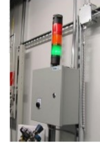
Gas alarms indicators in Cleanroom
