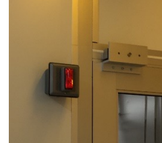
Gas alarms indicators in Cleanroom
